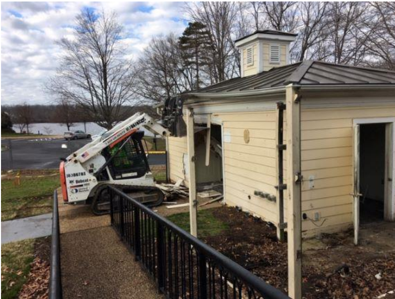
We then tore up the concrete patio over the old pool.
