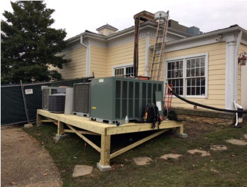
Old pool building used for extra refrigeration.
