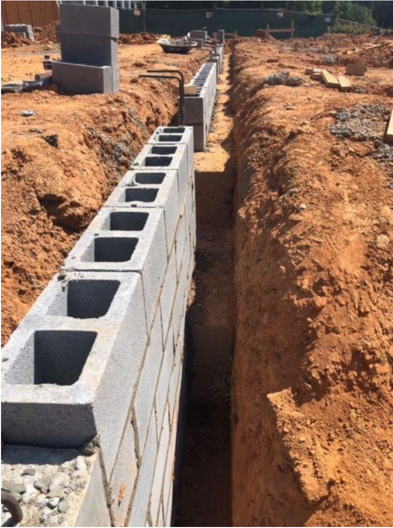
Groundwork has been completed and area ready for slab pour.
