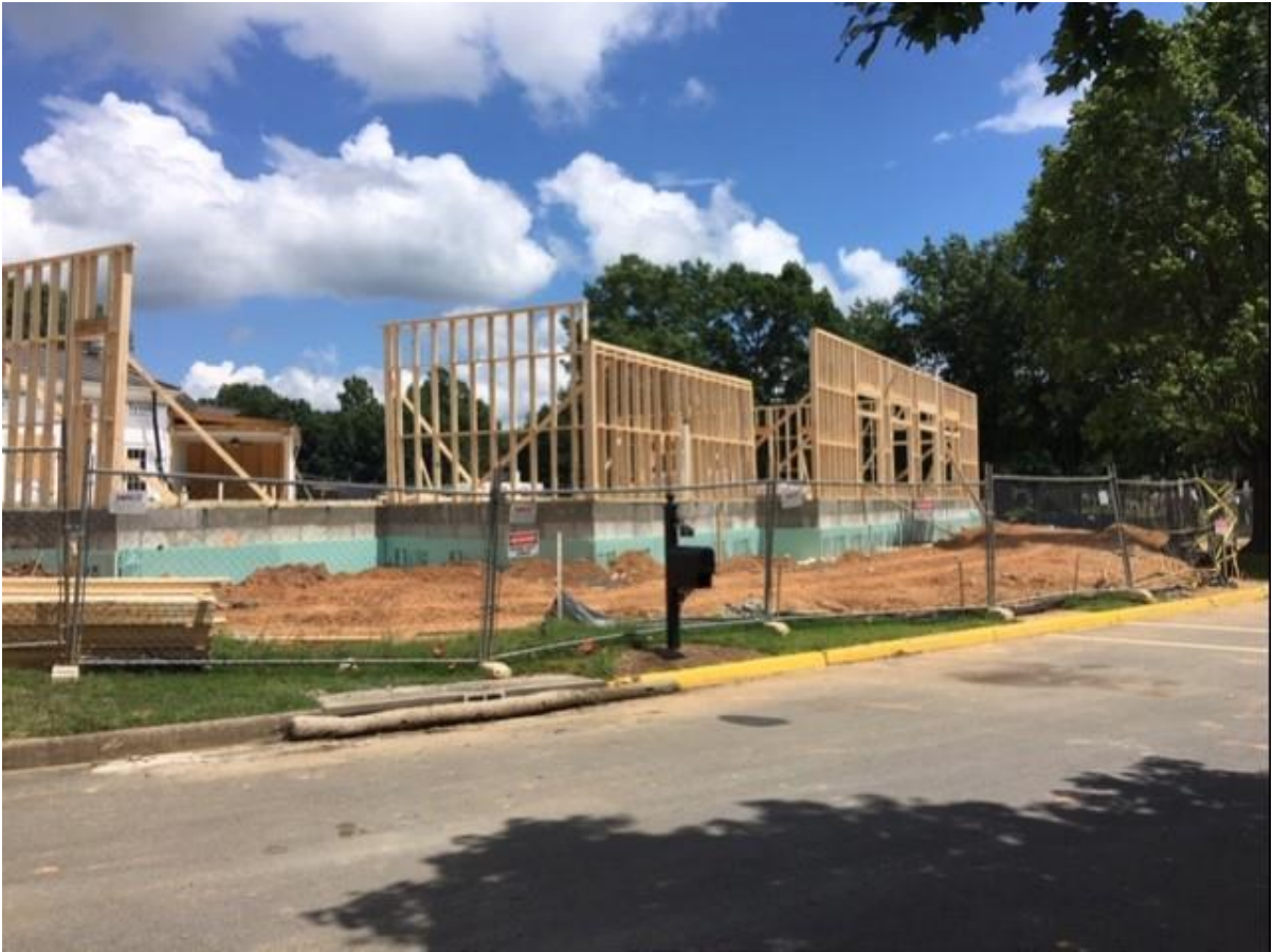
And largely finished!
