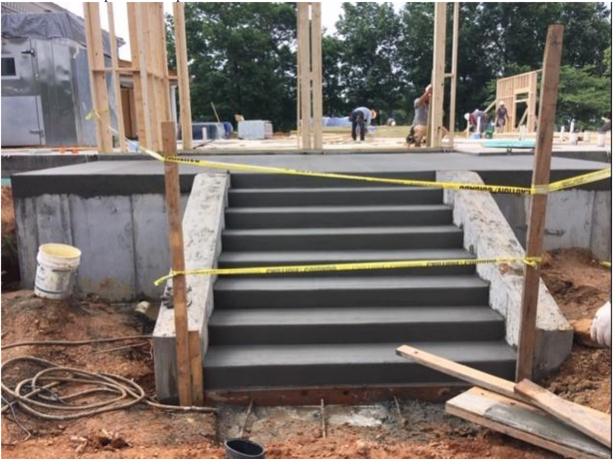
Framing was started
