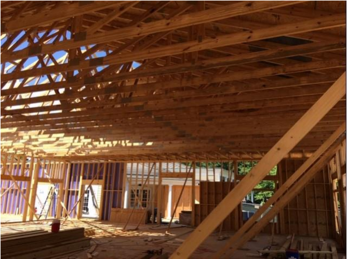
Roof was framed and prepped for shingles.
