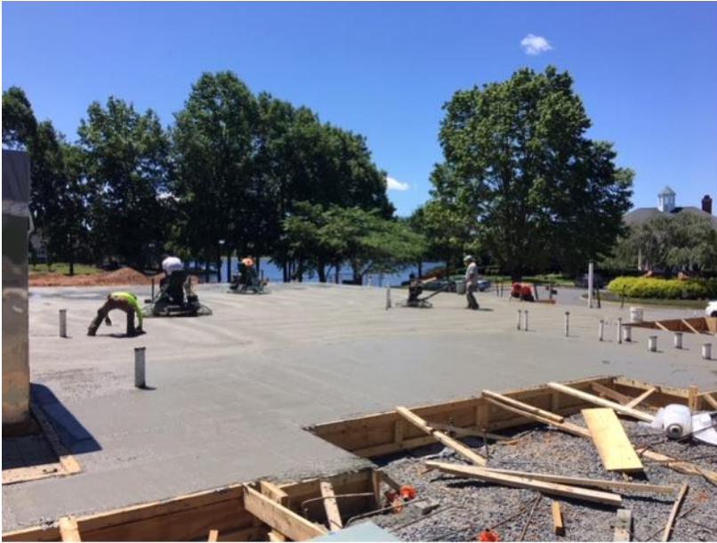
Front entrance steps were also poured
